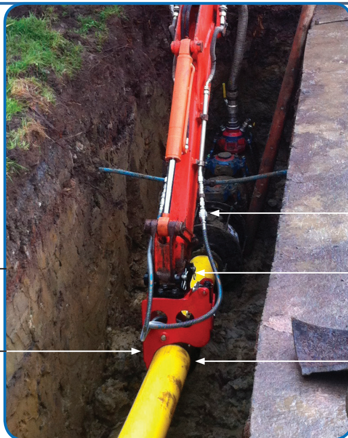
The Midi Pipe handler inserting 180mm PE, fitted with a Live Head for Live Mains Insertion
