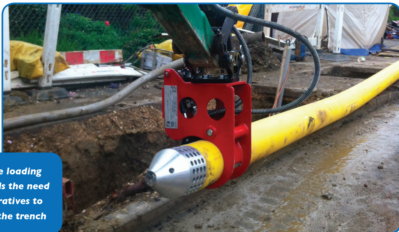
The Midi Pipe handler inserting 180mm PE, fitted with a Live Head for Live Mains Insertion
