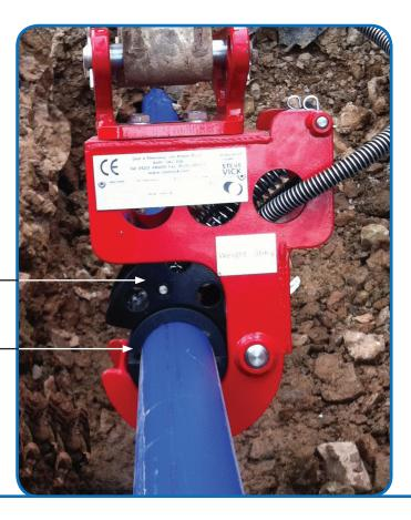
Hydraulically operated upper jaw
