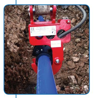
the hydraulic upper jaw clamps the pipe and inserts it into the host pipe using the hydraulic power of the excavator. Typical insertion speeds of up to 10 metres per minute can be achieved.
