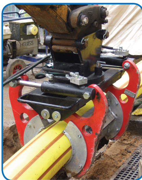
The 355 Pipe Handler, fitted with 250mm aluminium shells inserting PE into a host main
