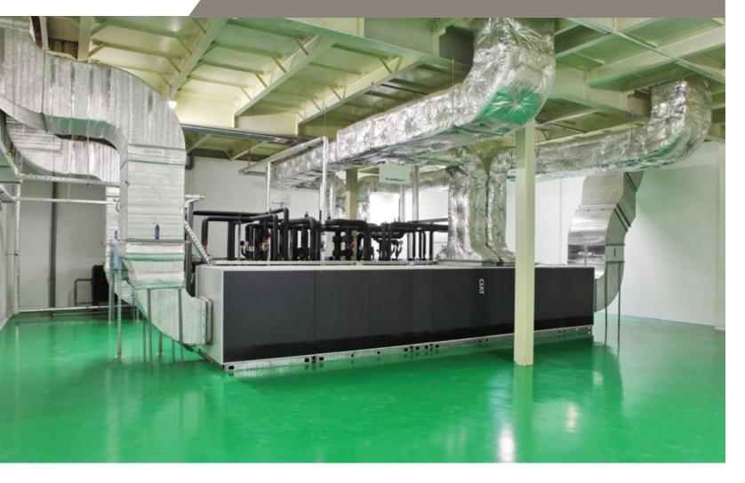
Protecting the flooring of Mechanical Equipment Rooms (MER) presents a unique set of challenges, with hazards including moisture, temperature, chemicals, and vibration. An effective coating system should deliver waterproofing that must not fail under these conditions. The PPG FLOORING MER System begins with Epoxy Primer, then builds with Epoxy Waterproofing Membrane and two-component Epoxy Top Coat to meet MER needs.
