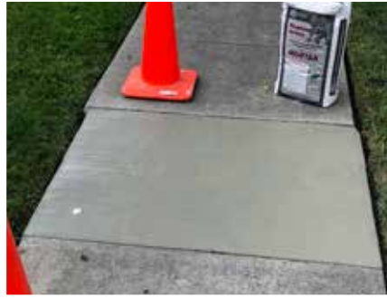
The area was resurfaced with Yeti Armor™ without deconstructing the failed surface.
