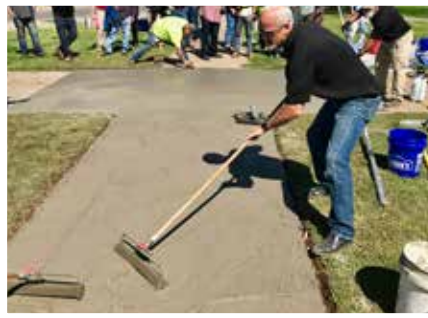
Applying Yeti Armor™ using Yeti's specialty rollers and tools.
