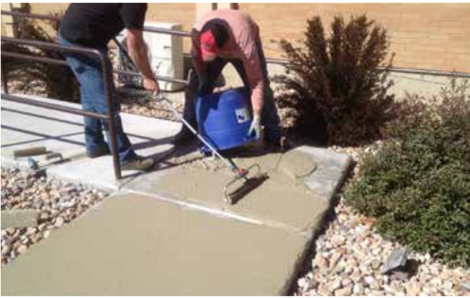
Yeti Armor™ rolled over pre-primed surface using 1/2" gauge.
