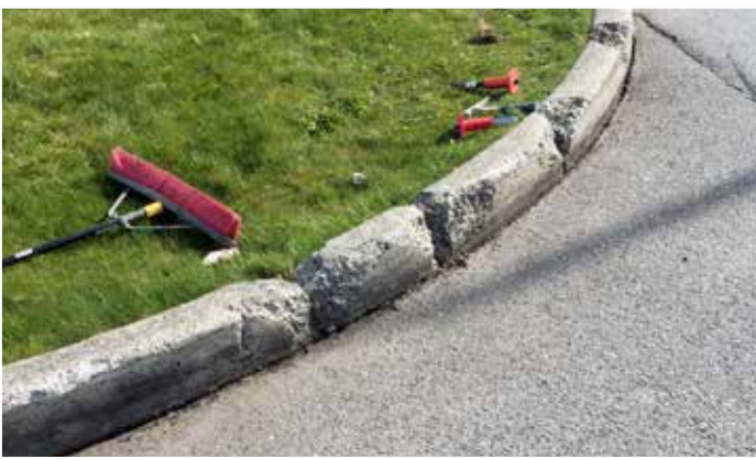
Damaged curb was repaired without deconstruction or forming.
