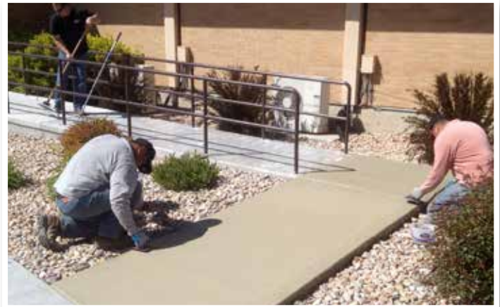
Overlay being finished using traditional finishing tools.
