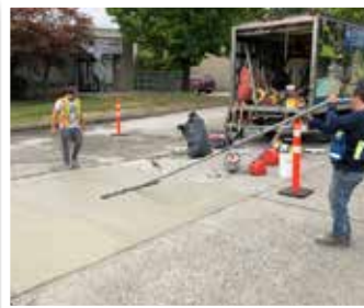
Place and finish Yeti Armor™ (see page 11 for recommended tools).
