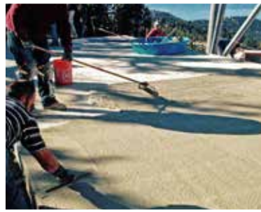
Yeti Armor™ applied with rollers and trowels.
