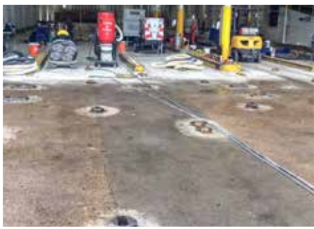
Existing surface cleaned, prepared and primed with Yeti Armor™ Overlay Primer.
