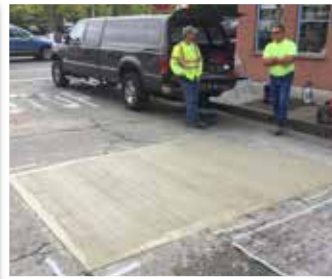
Repair completed with a broom finish.
