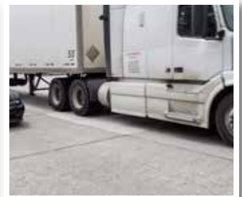
Roadway repaired for use in a matter of hours. Traffic volume in excess of a hundred trucks per hour.
