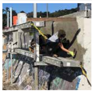
Severely degraded sea wall repaired three years ago using Yeti Armor™
