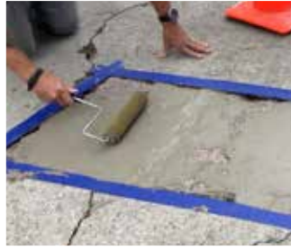
Cracks are pre-filled with Yeti Armor®
