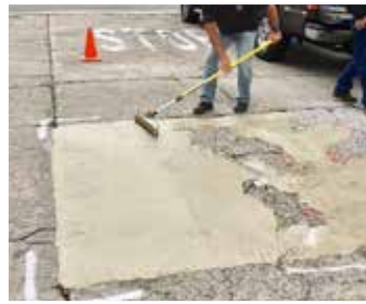
Yeti Armor™ being applied using a roller.
