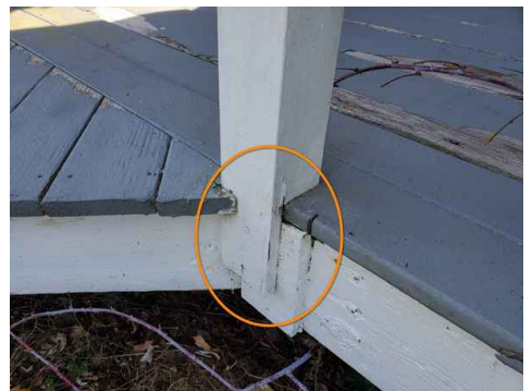
Posts notched for railings. Reduces strength of support posts. No longer notched.
