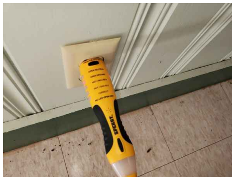
Basement Main Room
