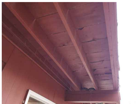
No ledger board attachment observed. Balcony is cantilevered, however additional support may be required for safety.
