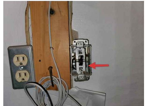
Basement Utility Room
