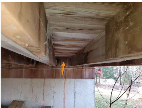
Missing ledger board and proper attachment to structure
