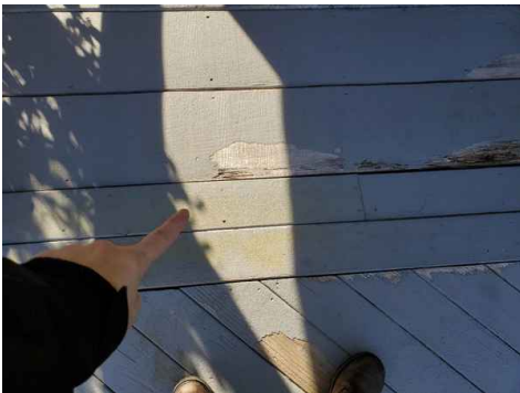
Board has deflection/movement when weight placed on board. Recommend replacement.
