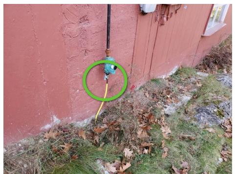
Valve along exterior
