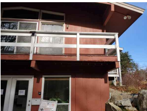
Cantilevered beams appear to be spanned at least 10-12 feet. This may require additional support and proper attachment to the structure
