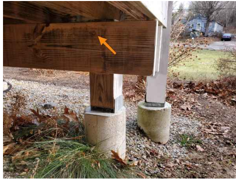
Thru-bolts at support posts and main girder
