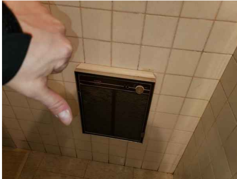
Basement Men's Bathroom
