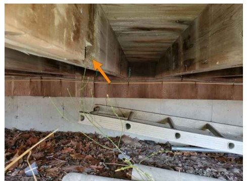
Multiple joists along deck appear to be sistered due to lack of proper support posts.
