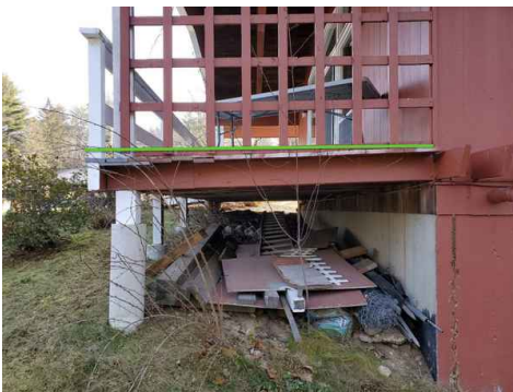
Settlement observed. Leaning outward.
