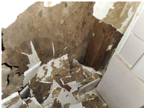
Basement Women's bathroom
