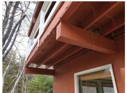
Span between cantilevered beams may need additional support posts.
