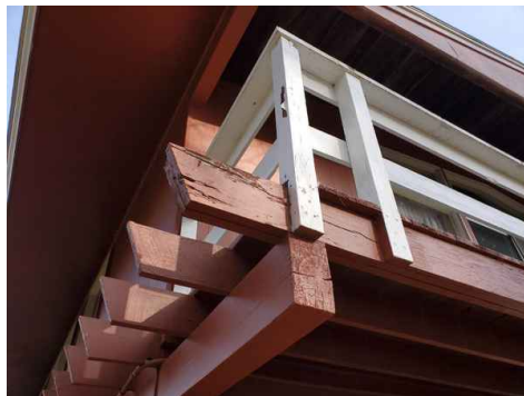
Notched support posts along railing.
