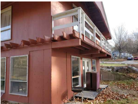
Horizontal guards along railing
