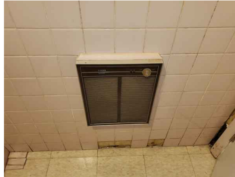
Basement Women's Bathroom
