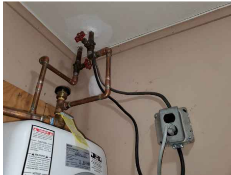
close proximity to water source. water heater
