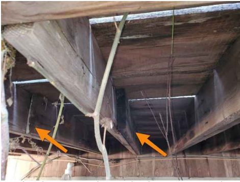
Multiple joists along deck appear to be sistered due to lack of proper support posts.
