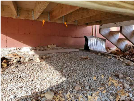
Joist hangers not properly secured with adequate fasteners. Ledger board attachment undersized (1/2" lag bolts minimum)
