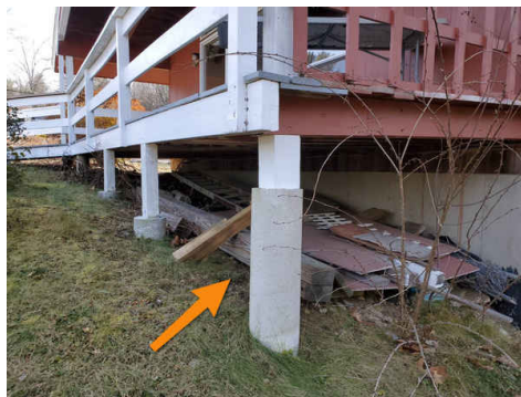
Poured footings exceed height recommendations above grade
