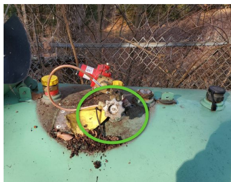
Valve at tank
