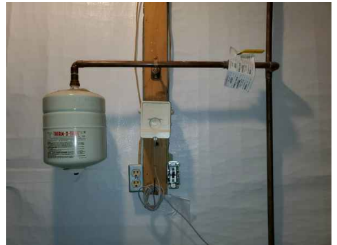
Close proximity to water source. main water valve
