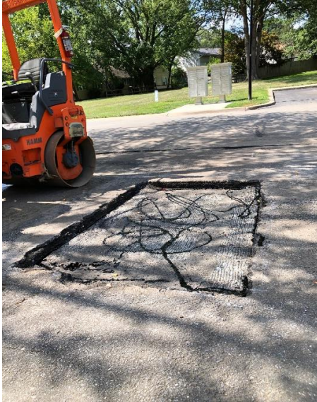
Repair Area Ready for New Asphalt
