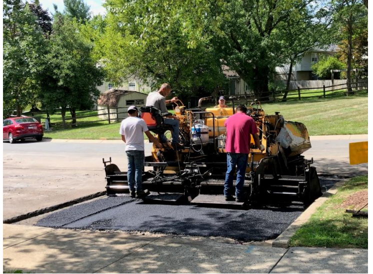
Paving in Progress in Repair Area
