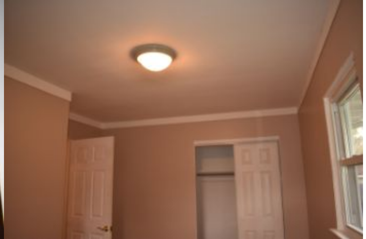
Walls and ceilings were in serviceable condition. No major deficiencies noted.
