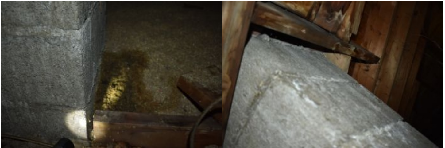
Chimney flashing is actively leaking
