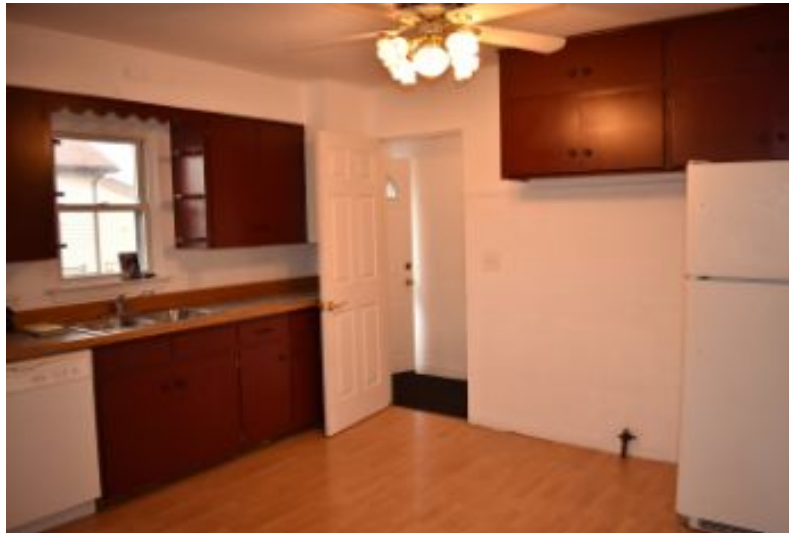
No major deficiencies observed on kitchen cabinets.
