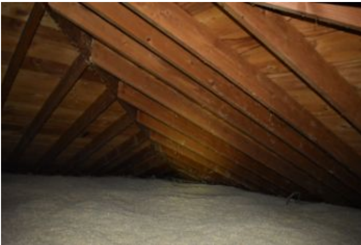
Attic structure appeared to be in serviceable condition.
