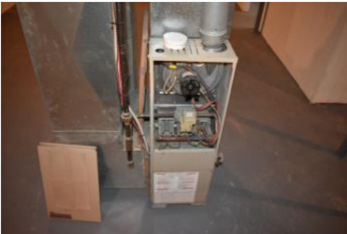
Fuel Furnace: Last service date is over one year ago, or is unable to be determined. Although this unit appears to be operating properly from controls, the inspector recommends further evaluation/cleaning/adjustments by a qualified heating contractor.
