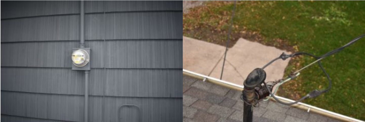
There is an overhead service drop noted.
