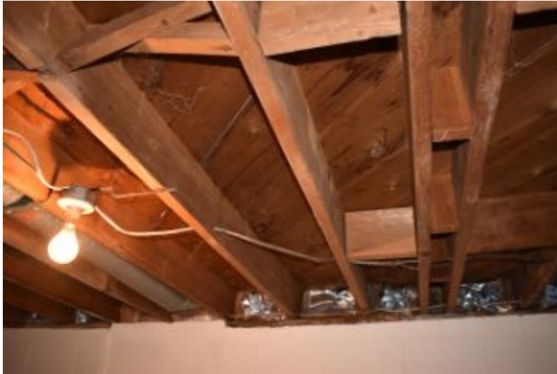
Planked subfloor noted.
