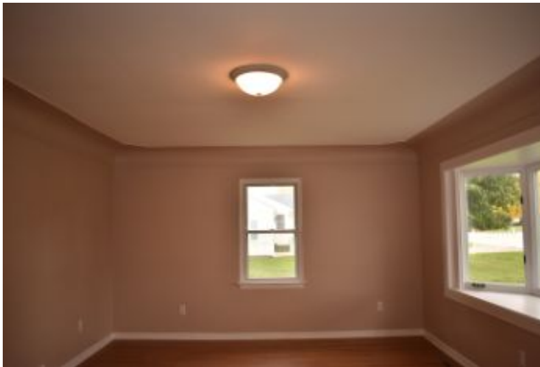
Walls and ceilings are in serviceable condition. No major deficiencies noted.
