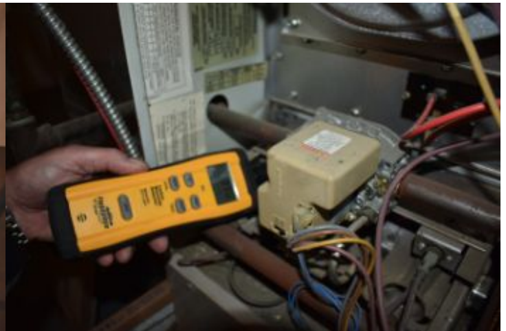
Elevated ambient Carbon Monoxide (CO) noted during tial operation. Do not use furnace until it is evaluated by a qualified heating contractor.
