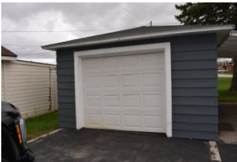
Door(s) appeared serviceable at time of inspection.
