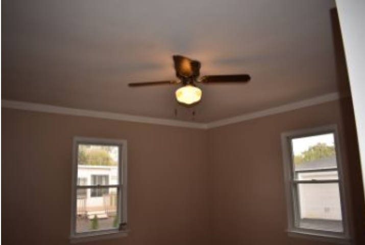
Walls and ceilings were in serviceable condition. No major deficiencies noted.
