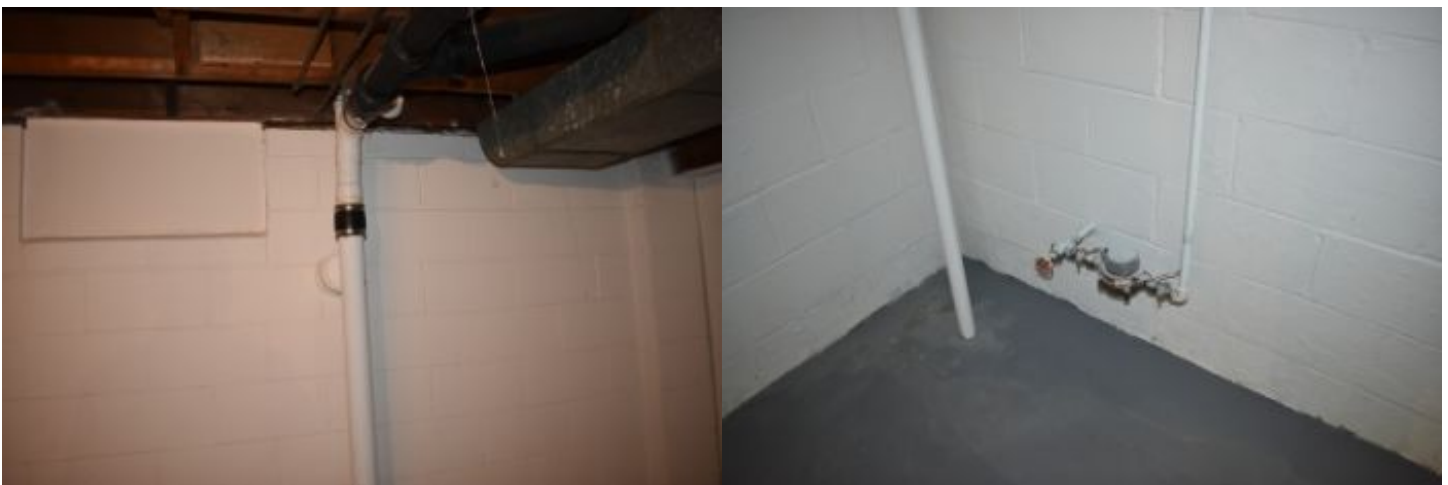
Cast iron waste and vent pipe noted.
