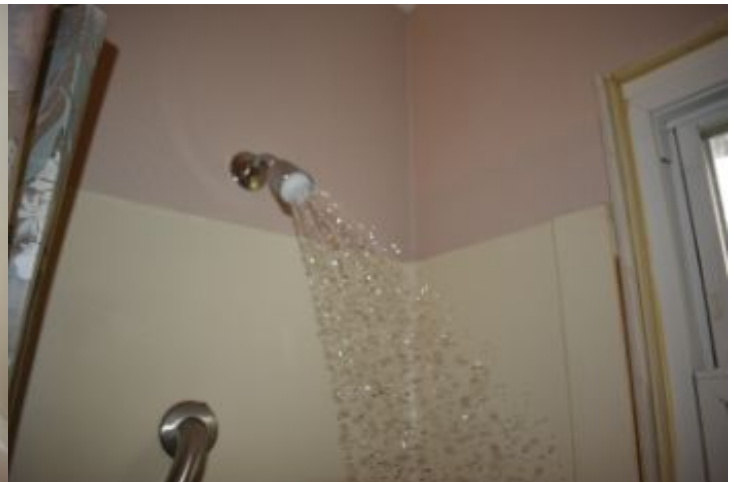
Combination tub/shower noted.
