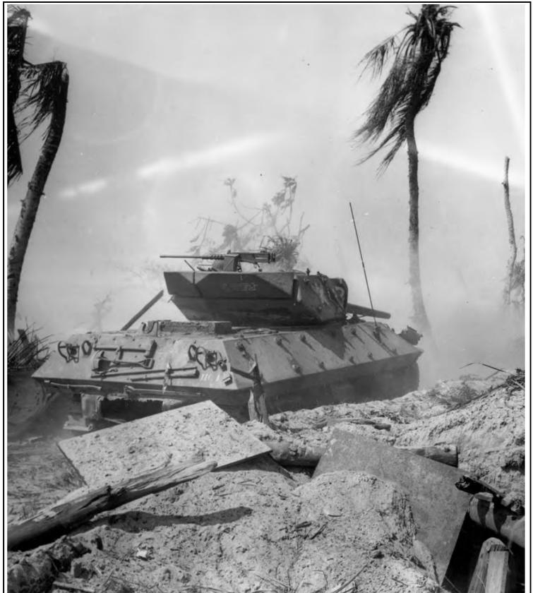
GUN MOTOR CARRIAGE M10, used to blast pillboxes on Kwajalein. This weapon, called a tank destroyer, was mounted on the medium tank chassis and had a 3-inch gun M17 in a semiopen turret, and a .50-caliber machine gun at the rear of the turret for protection against low flying planes. Six days after the main landings had taken place, Kwajalein was in U.S. hands.
