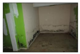
Mold: This usually occurs in the basement. Also look for the bottom half of the drywall missing (like in the second picture below). This virtually always means mold was torn out. Mold isn't hard to remove, but the key is to find out where water is
