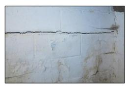
**Foundation Movement:** Anything over four inches should probably be braced or have "dead men" added. Much more than that and the wall might need to be pushed back, which is very expensive. (Pro tip: If you can't tell how much the wall has moved, go outside and run you finger along the bottom of the siding. It should go about to your knuckle. But just running it along the foundation wall should give you an idea of where and how much the wall has moved.)
