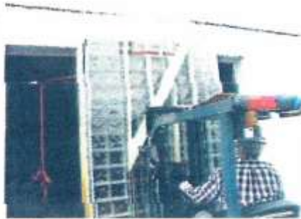
Carefully align panel on all sides before moving into framed opening.
