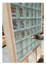
11. Using a rubber mallet, tap the vertical glazing strips into place.
