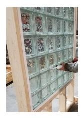
12. Using a rubber mallet, tap the vertical glazing strips into place.
