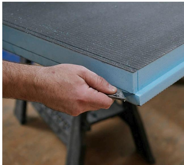
**EN** A wedi shower base can be cut to size using a circular saw with standard carbide blade. You can remake the 1/2 in. x 1/2 in. perimeter channel by cutting through the cement surface using the circular saw set to cut 1/2 in. deep. You can use a circular saw or a sharp utility knife to cut the new channel 1/2 in. wide through the blue exposed foam side. Clean the new channel and the base and remove all saw dust and loose particles.
