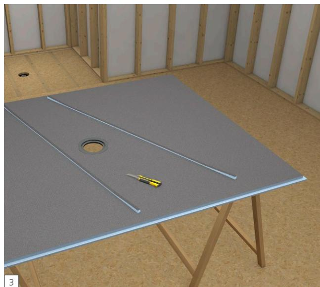
**EN** Once the base is cut to size, you want to dry fit the base and remake the perimeter channels on all sides which will connect to wedi wall panels. The perimeter channel must be 1/2 inch wide and between 1/2 inch and at minimum 3/8 inch deep. The minimum thickness of the horizontal part of the perimeter channel bottom must not be less than 1/4 inch.
