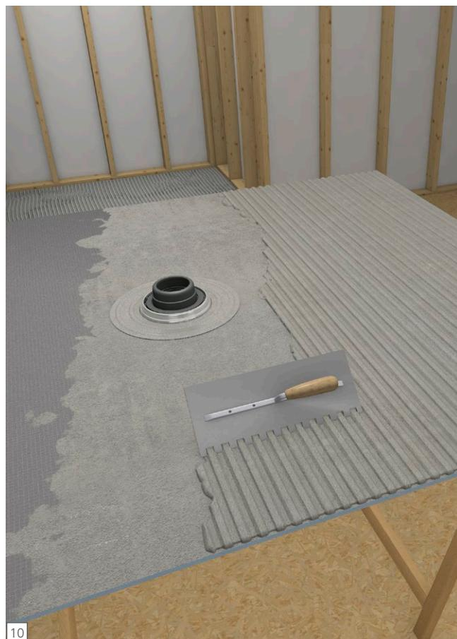
**EN** Trowel the thinset on the rear side of the Fundo again using a 1/4 in. x 1/4 in. notched trowel. Flat trowel the thinset over the entire product's cement surface, then comb through thinset bed creating channels pointing in same direction as applied on subfloor. If a 1/2 in. square notch trowel was used to apply thinset to the subfloor, you want to apply only a flat skim coat of thinset on the rear side of the Fundo.
