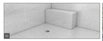
5. Start tiling immediately once sealant and thin set tile adhesive is dry to the touch.
