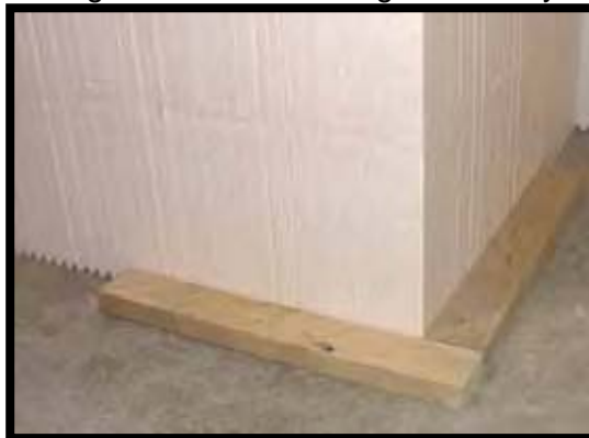
Fig 6.1 2" x 4" (5.2 cm x 10.2 cm) kicker plate fastened to concrete floor, footing, or slab.
