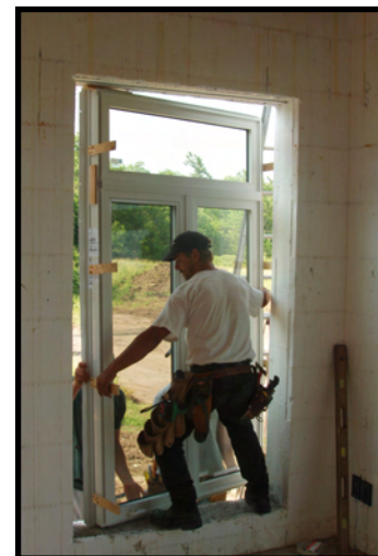
Fig 10.1 Sample of window installation
