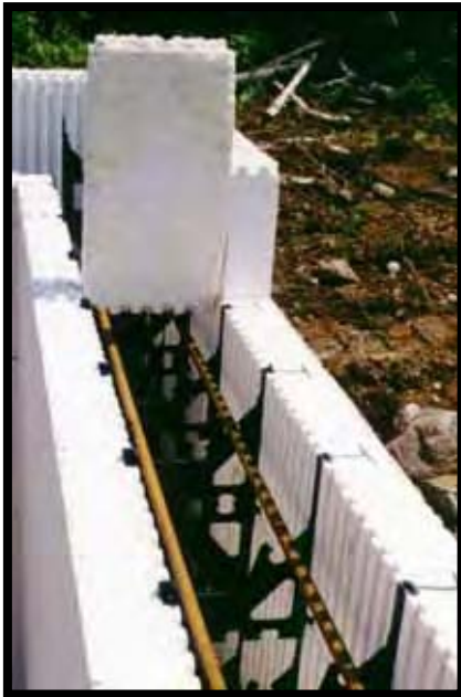
Fig 11.2 Sill steel installed as wall is constructed
