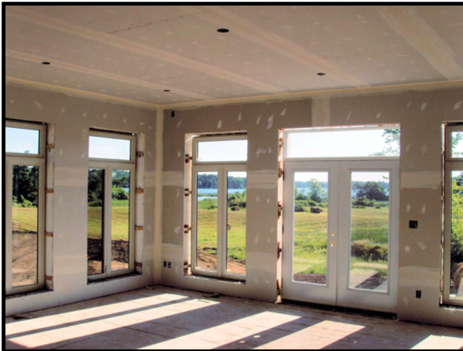
Fig 10.2 Installed windows with IntegraBucks and IntegraHeaders
