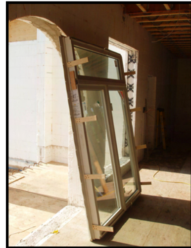
Fig 10.3 Windows ready to install
