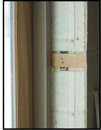
Fig. 10.1 Reduce installed costs. Improve energy efficiency- "stucco friendly" one material external substrate.
