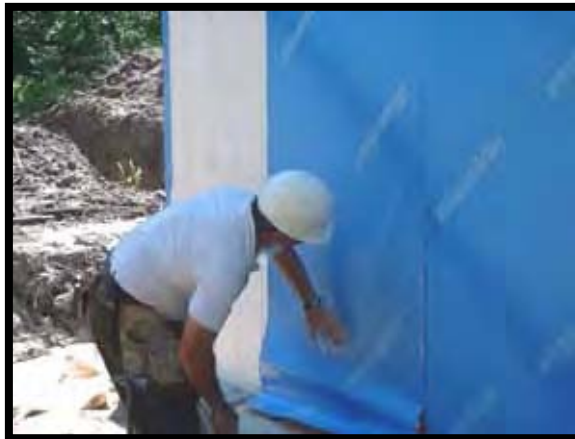
Fig. 19.1 Peel and stick waterproofing membrane (below grade application)
