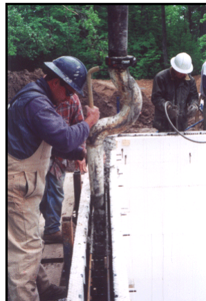
Fig. 17.2 Filling IntegraSpec ® Wall using Pump Truck boom with double 90.
