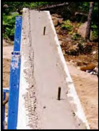
Fig. 17.4 Anchor bolts at top of wall for anchoring floor / roof sill plate
