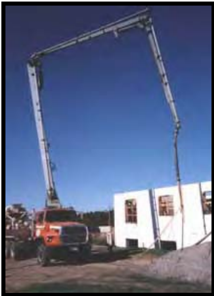
Fig. 17.1 Concrete Pump Truck with boom.
