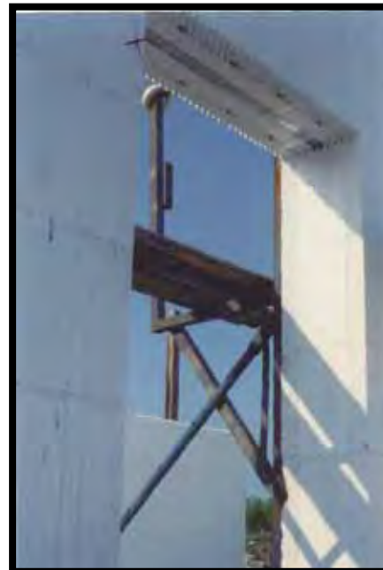
Fig. S-8.1 IntegraHeader (top) & IntegraBuck (sides) (optional steel (header) channel shown)
