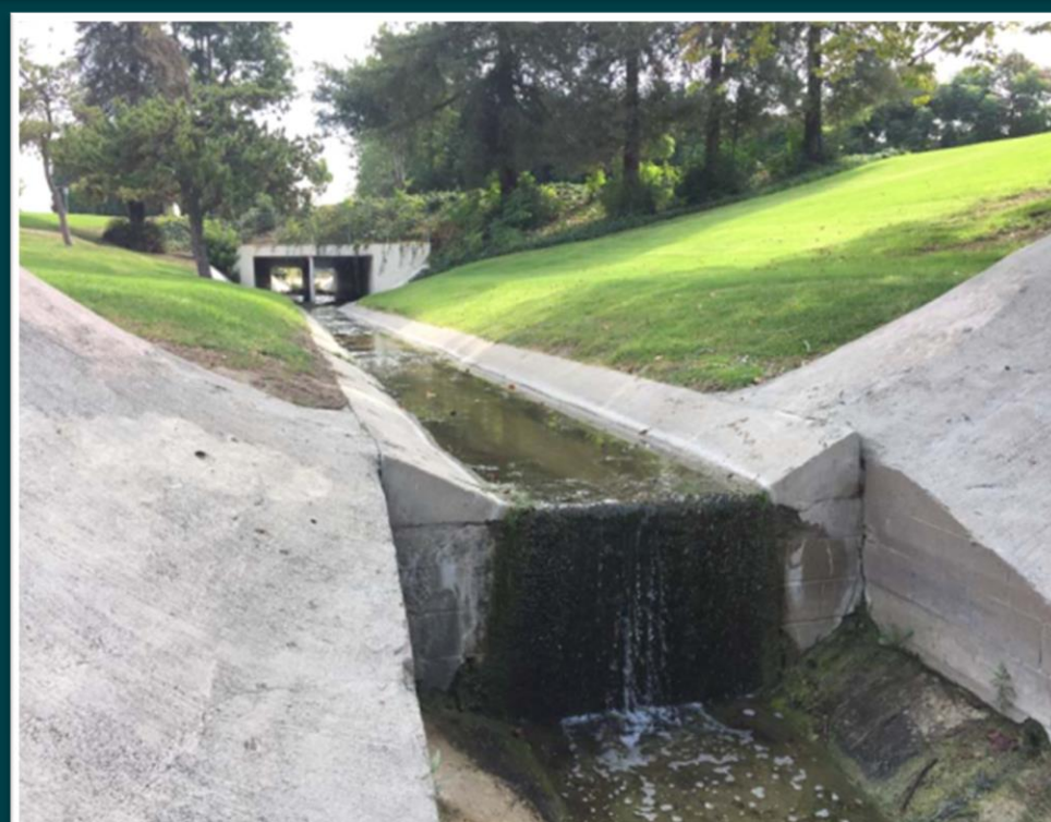
Existing Concrete Channel
