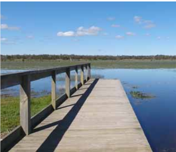
5.12 Tae Rak Visitor Experience Area: Jetty and boat ramp
