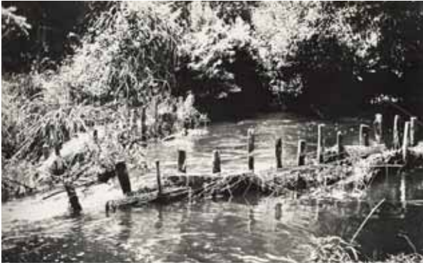
3.13 Eel weir (pa tuna) named Ruataniwha, on the Hokino Stream. The pā tuna (eel weir) was a common device for catching eels in rivers, streams and the outlets of lagoons and lakes. Weirs were used in autumn, to catch eels as they headed downstream to spawn in the sea. Fences in the water guided the eels into a net and then into a hinaki (eel pot). Pā tuna were useful when rivers were in flood or flowing heavily.
