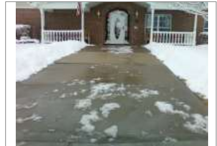
The sidewalks leading out of Brookdale/Emeritus at Denver facility were icy and posed a risk to residents and visitors.
