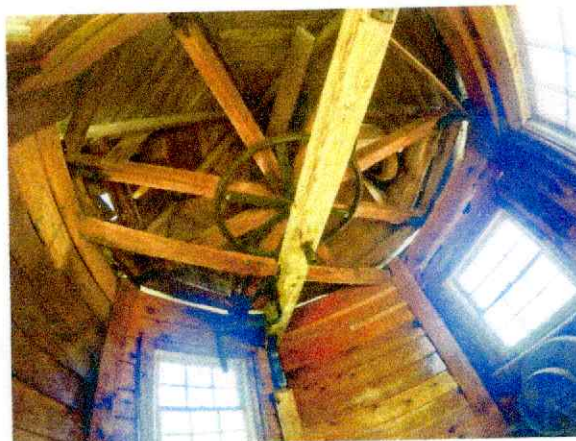
Inside Roessler windmill's second floor featuring the winch mechanism used to turn the cap. (2018 - Photo Liz McCafferty)
