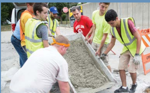
Students embed electrodes linked to a data acquisition system into “smart” concrete.
