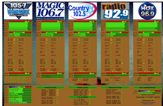
Fig 4 This large computer screen is programmed to show bar graphs of plate voltage, plate current, forward power, HD Radio forward power, room temperature, and transmission line pressure as well as hundreds of status values all at a glance
