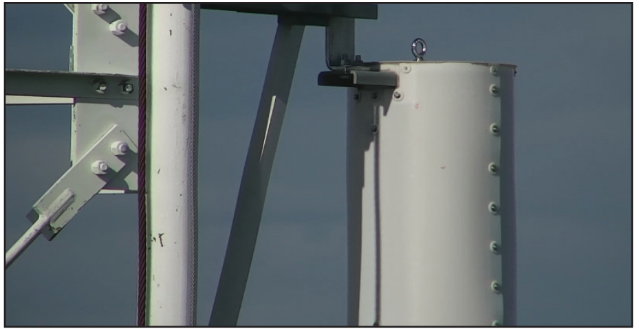
Close up inspection of a side mount UHF TV Antenna
