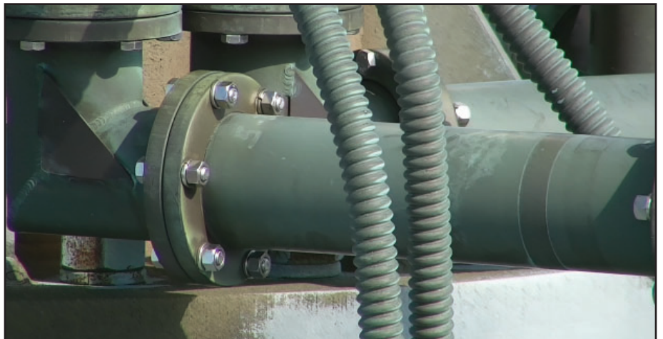
Examining the flange bolts at 1,000 feet above the ground
