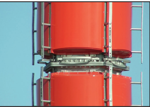
Close up of the joining section of a top mounted UHF TV antenna
