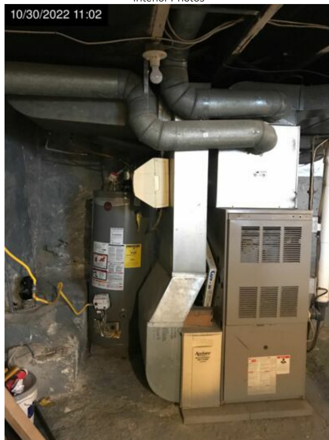
HVAC Unit Interior Photos
