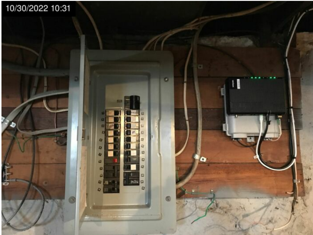
Electrical panel Interior Photos
