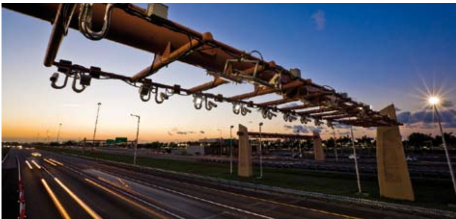
☛ By 2012, traditional toll plazas will be eliminated and gantries equipped to read SunPass signals will be in place on all MDX expressways. There will also be the alternative to join a video tolling program
