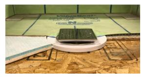
Installed in a thin-bed method shower with ValueSeal® waterproofing sheet membrane, and ProBase® II Multi-Slope Base.
