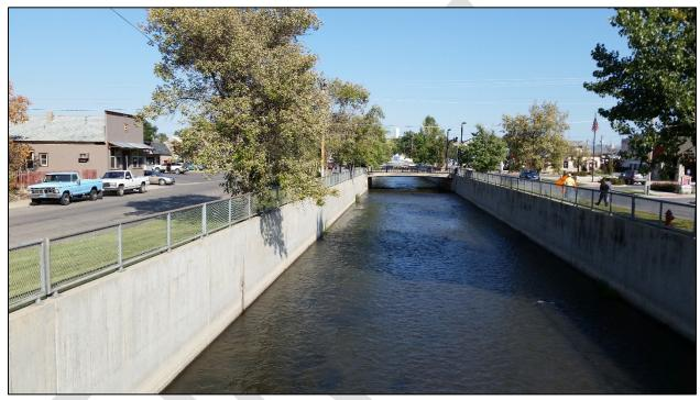
Figure 7. View looking east at the concrete-lined channel portion of Little Goose Creek
