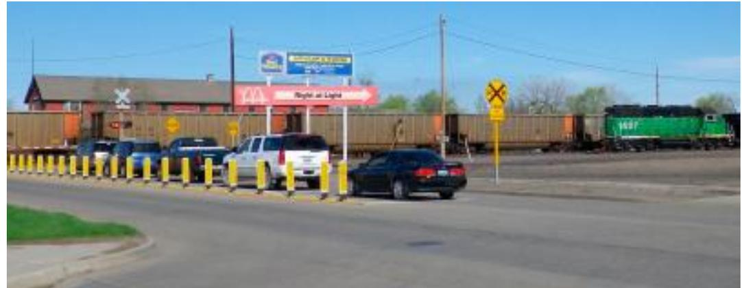
Figure 3. Non-traversable median at train crossing
