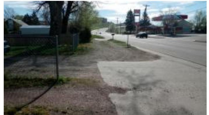
*Vertical displacement of sidewalk and tripping hazard, missing sidewalk links, and deteriorating concrete*
