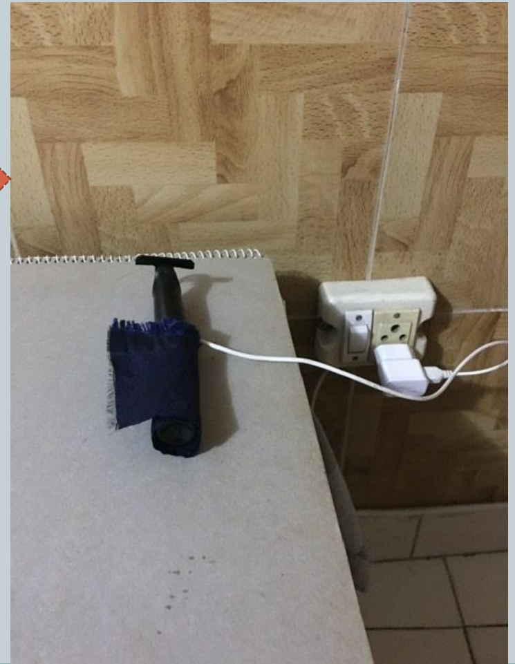
Electrically Heating Oil
