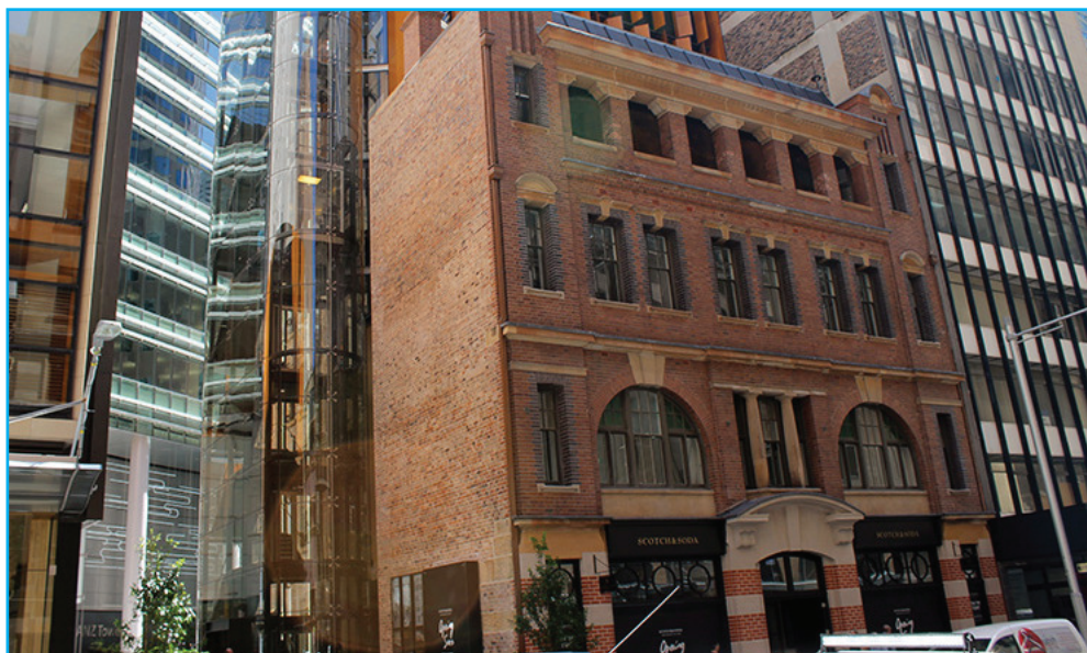
The glass lift and stair contrast the old brick wall nicely, while providing a modern entry
