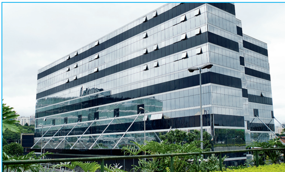
Renovated in 2007, ROI time for this university's Jets™ system was just 15 months
