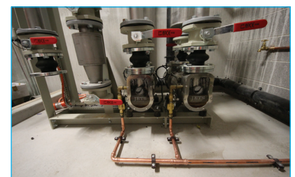
The Jets™ 130MBA vacuum unit used by Melbourne Water features two 65MBA pumps.
