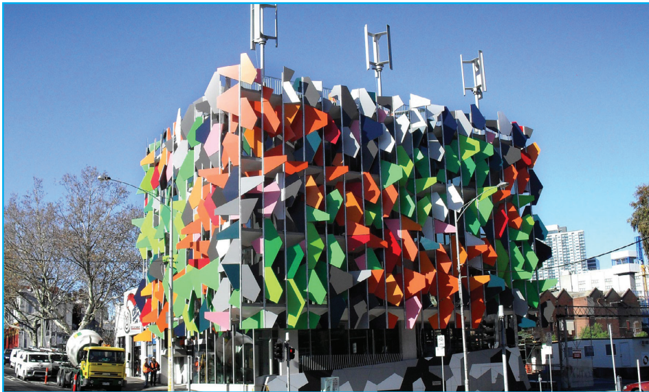
The characteristic colour panels are designed to let daylight in but keep sun heat out
