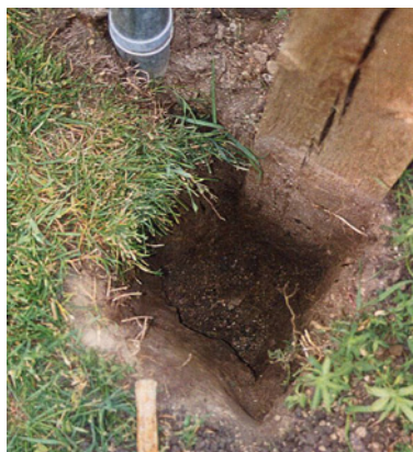
Fig. 2 – Destroyed monument at fence corner
