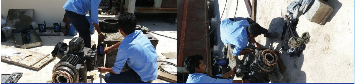
Jami Al Adliya – Compressor Overhauling
