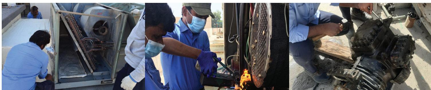
Jami Al Ghudaibiya – Ducting Works
