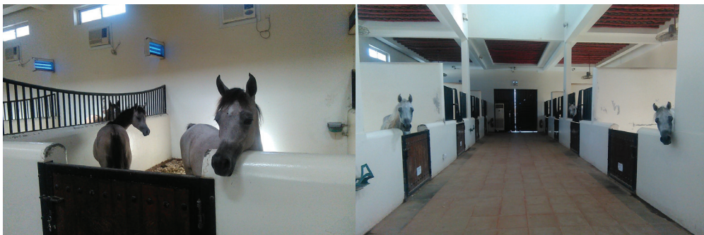
New AC Installation in Horse Stable – Jasra
