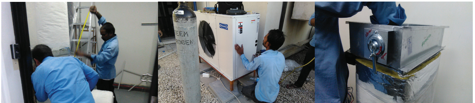
BIBF – Mechanical Works
