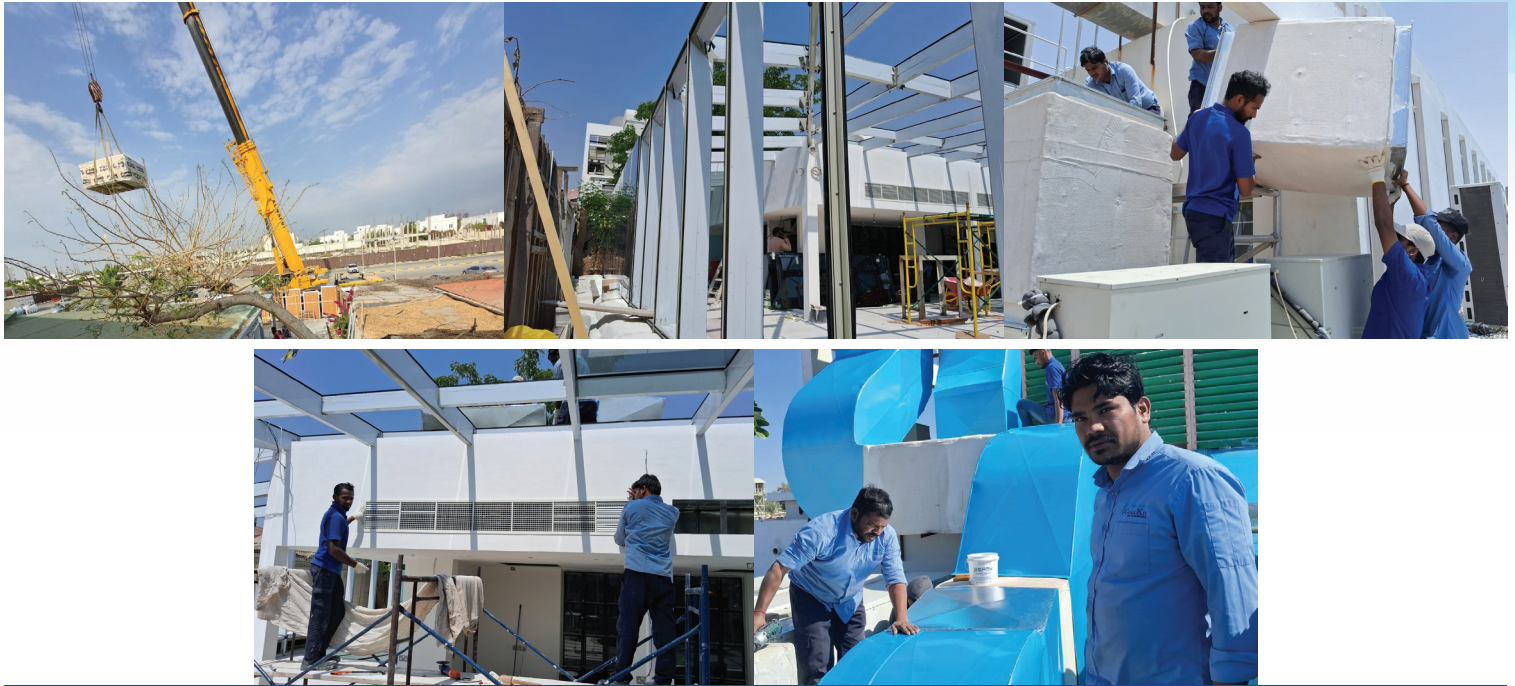
Villa Mamas Project – MEP Works
