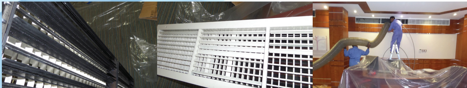
Civil Service Bureau – Duct Cleaning
