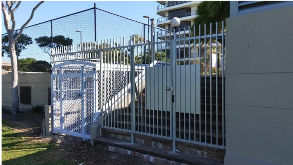
Figure: new eastern gate and fence.
