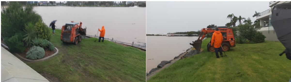
Figure: Mark supervising repairs to the sink hole in the rain
