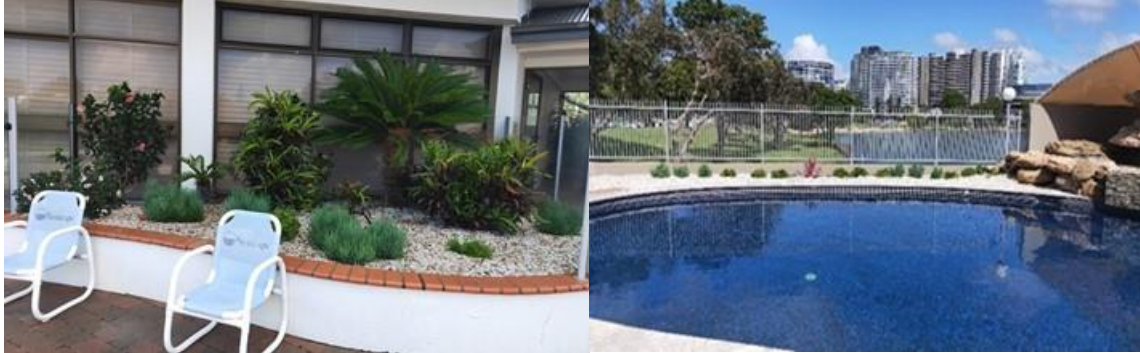
Figure: Removal of palms that were damaging the walls and membrane and replanting with suitable plants with non-evasive roots.
