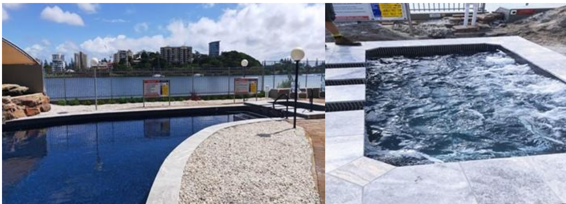
Figure: New coping, new tiles below the coping providing a modern look.
