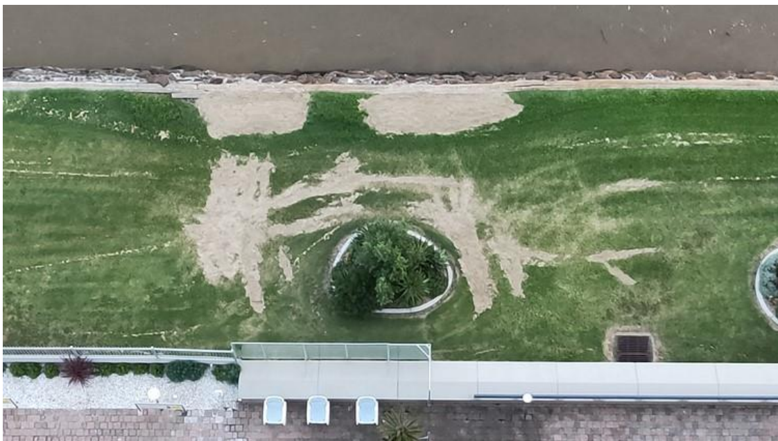
Figure: Completed repairs to the sink holes
