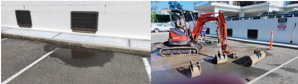
Figure: Lower carpark sink hole repair
