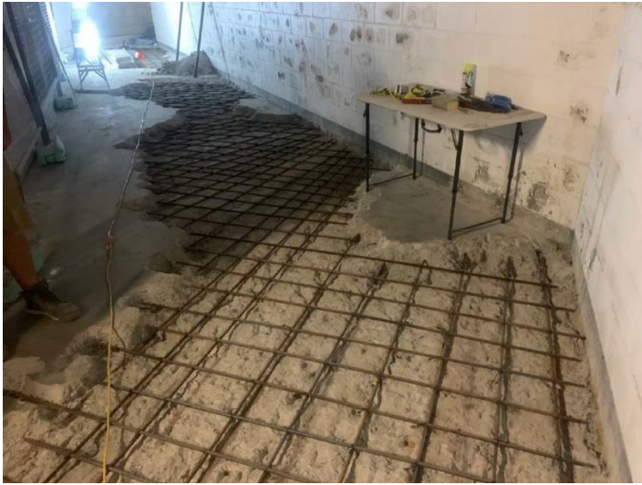
Figure: Basement spalling bike rack area.
