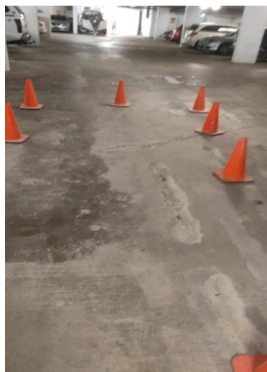
Figure: Areas of Concrete spalling (cracking concrete) have been treated and repaired.
