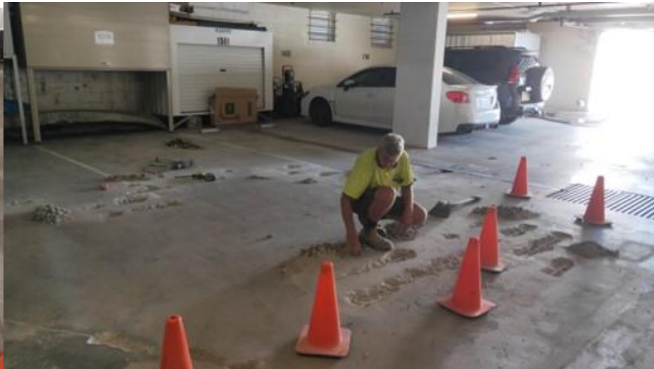
Figure: Areas of Concrete spalling (cracking concrete) have been treated and repaired.
