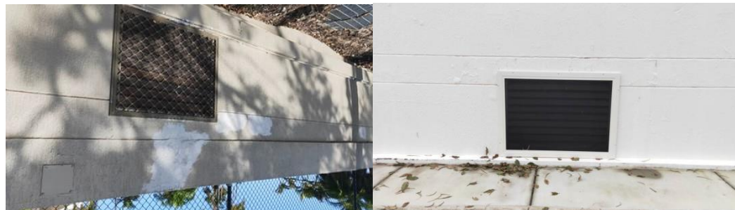
Figure: Grills replaced.
