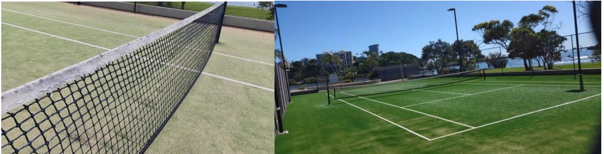
Figure: Tennis Court upgrades with repair of slab crack and waterproofing.
