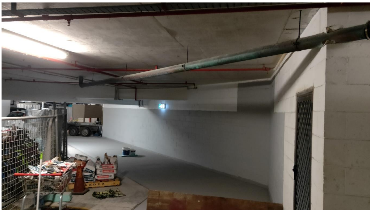
Figure: Process followed for the remedial work.
