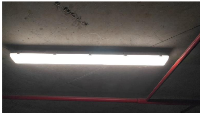
Figure: New basement lights replacing faulty lights.
