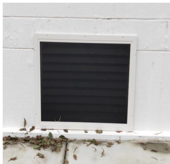
New security screens
