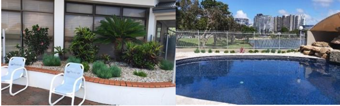
Figure: Removal of palms that were damaging the walls and membrane and replanting with suitable plants with non-evasive roots.
