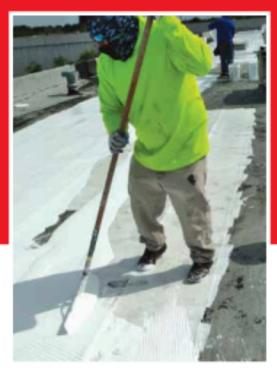
water damages. These areas were removed and replaced with ISO board and covered with modified bitumen. 13 areas in total were repaired. We also installed crickets to assist in water flow to the scuppers and gutter systems. We were then able to provide a 15 year warranty with the silicon product.
