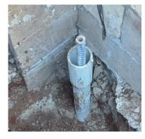
Condor soil stabilizer was injected into the soil under the slab on grade using these tubes & hoses (Right photo)
