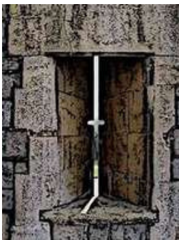
Arrow Loop Inside View
