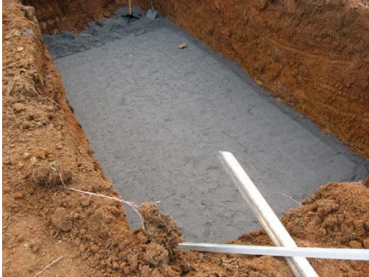
Photo 4.1.4-Bedding material prepared for setting the tank
