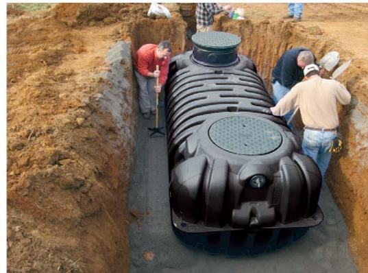
Photo 4.1.6-Spreading & compacting of backfill material
