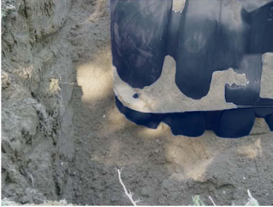
Photo 4.1.7-Proper support for vessel
