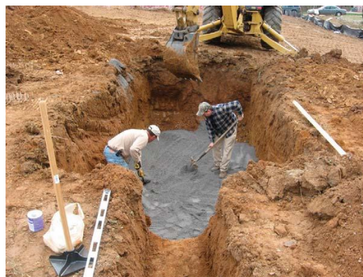
Photo 4.1.3-Bedding being spread and compacted
