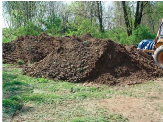
Photo 4.1.10-Example of backfilling material
