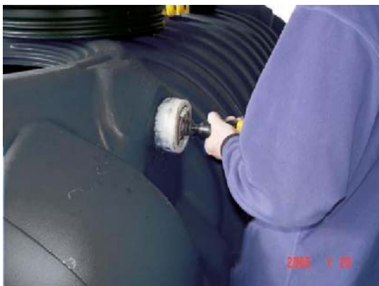
Photo 4.1.1-Drilling of inlet and outlet holes
