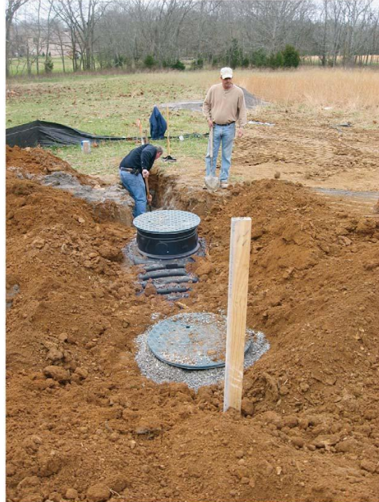
Photo 4.1.12-Example of complete backfill
