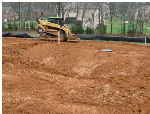
Photo 4.1.14-Example of final grading
