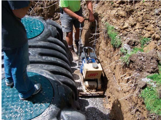
Photo 4.1.8-Example of mechanical compaction
