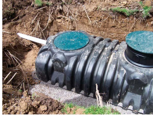
Photo 4.1.9-Uniform level distribution of material
