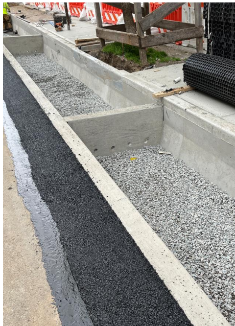
STONE HEADERS CHECK DAMS
