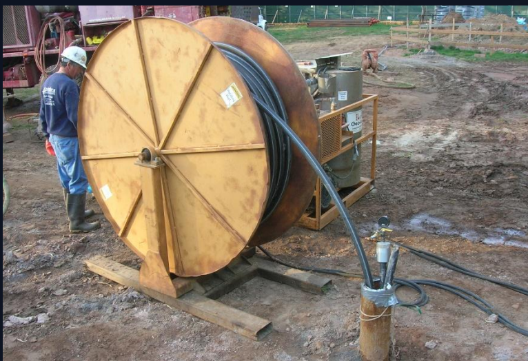
Grouting Process – Tremie Pipe Hose Reel
