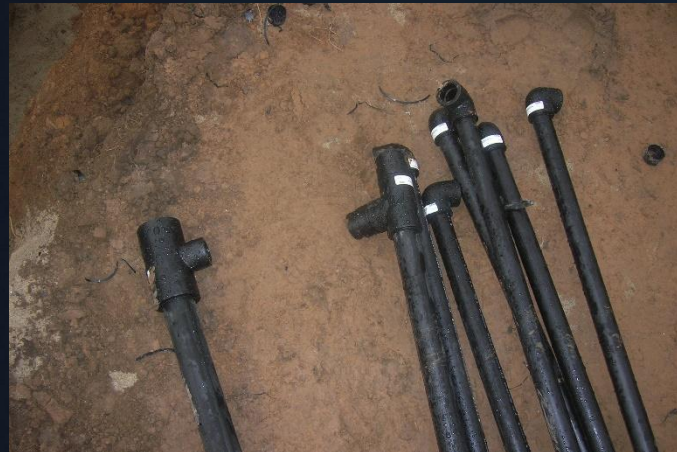
Horizontal Pipe Fittings Pre-assembled
