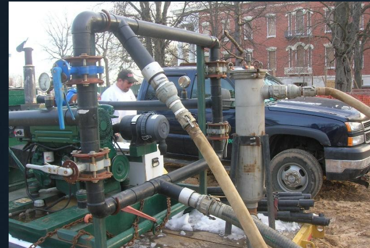
Final System Flush, Purge, and Pressure Testing
