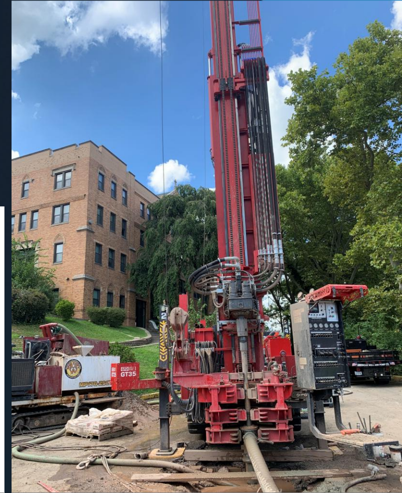
Test Bore Installation
