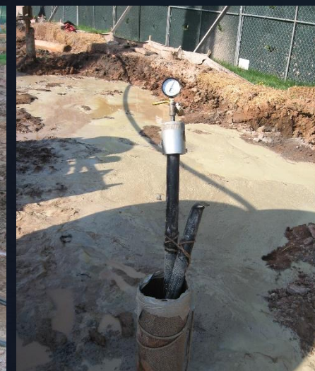
Grouted Loop/Pressure Test
