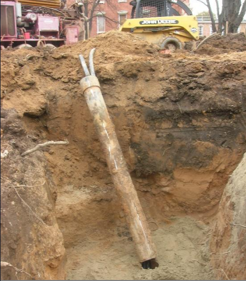
Borehole Casing Cut Down to Trench Bottom
