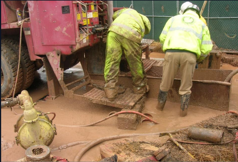
Drilling In Progress
