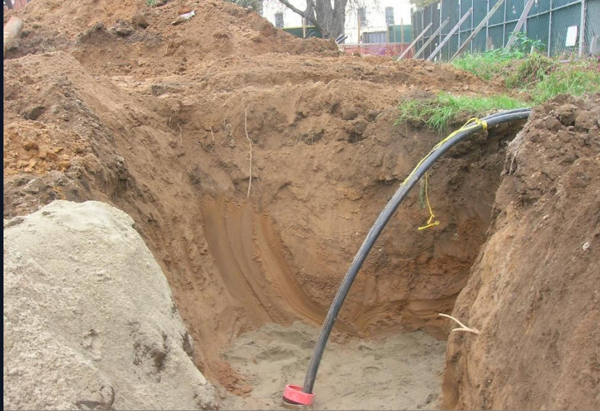
Protective Lip Installed on Casing
