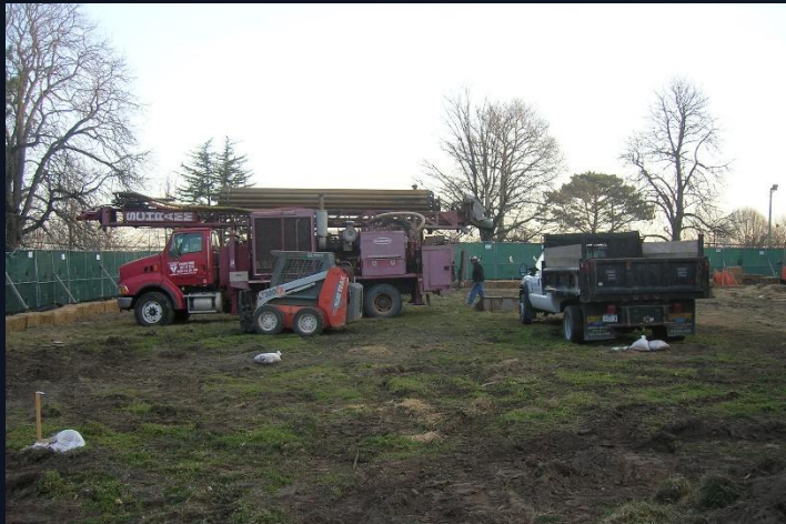
Drill Rig and Support Vehicles
