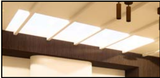
CONTINUOUS BEAMS THROUGH SKYLIGHT
