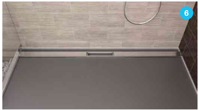
Step 6. Attach the grate to the channel. With the sliders positioned correctly, place the grate over the base and make sure the grate looks centered in the shower, adjust accordingly.
