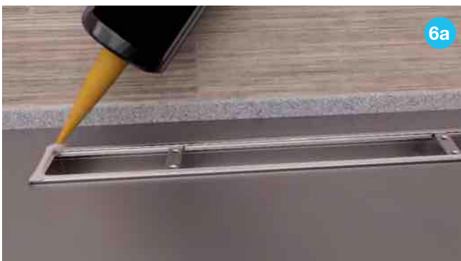
6a. Once grate and slider position are verified, apply sealant around the top edge of the base and thin-set to the bottom of the grate, or remove the paper backing from the sealant tape.
