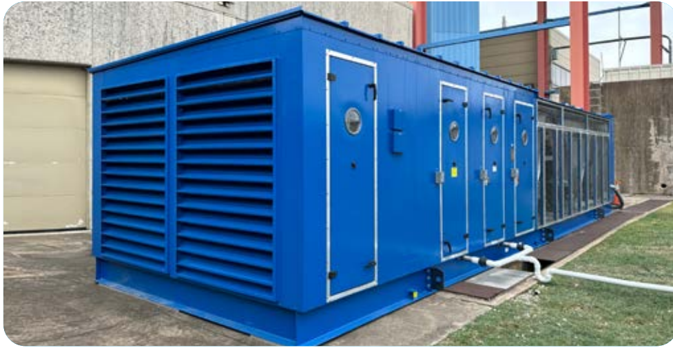
SkyH2O Maximus 4260 commercial-scale atmospheric water generator for modular water production.
