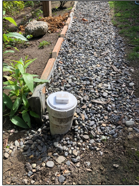
FIGURE 2: Well-maintained trench.
