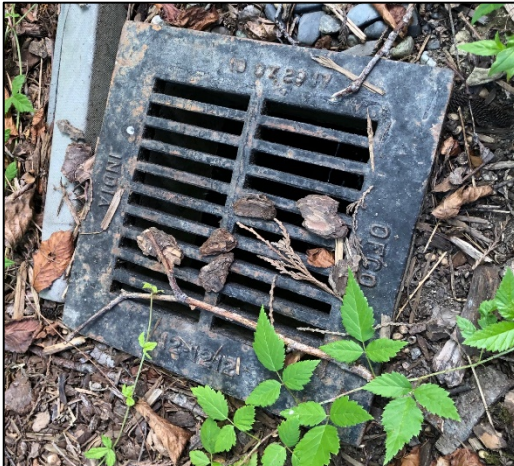
FIGURE 3: Grate in need of clearing
