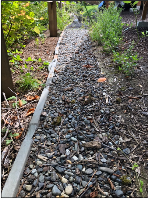
FIGURE 1: Trench in need maintenance
