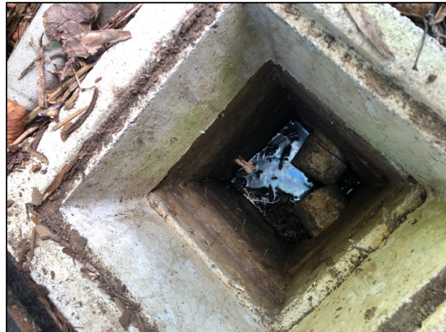
FIGURE 4: Clear drain with mild sediment
