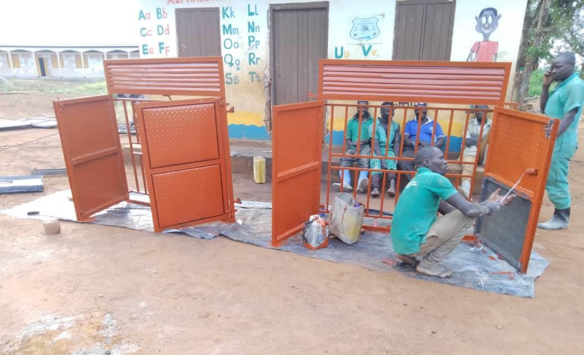
Steel was used to make the windows and doors and then these were painted
