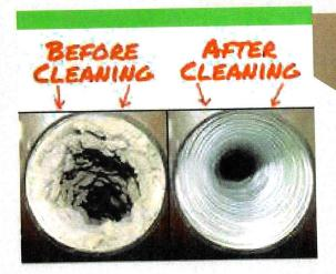
Clogged dryer vents, ducts, and filters are the main causes of dryers catching on fire.
