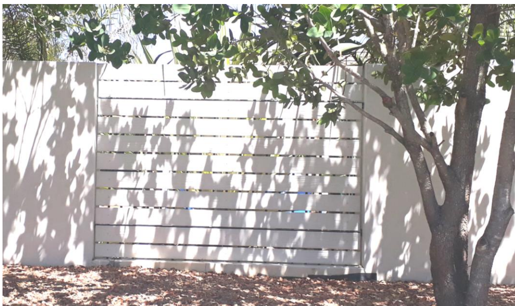
Nutec “Handi-planks” fibre cement closers (with visible gaps for increased visual permeability)
